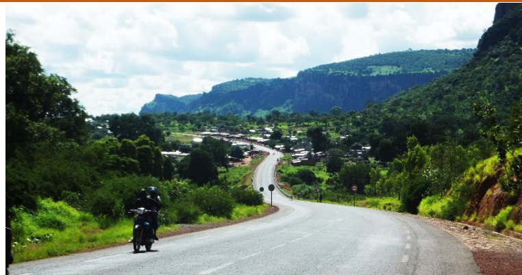
A SECTION OF THE SARAYA-KITA REGIONAL ROAD
