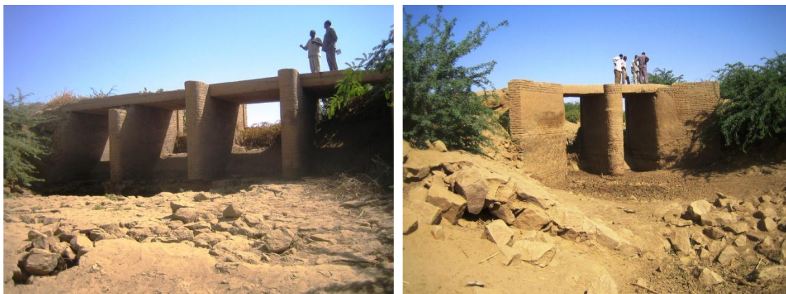
Cross-regulators along main canal in Kassala Block © IFAD/Olaf Verheijen
